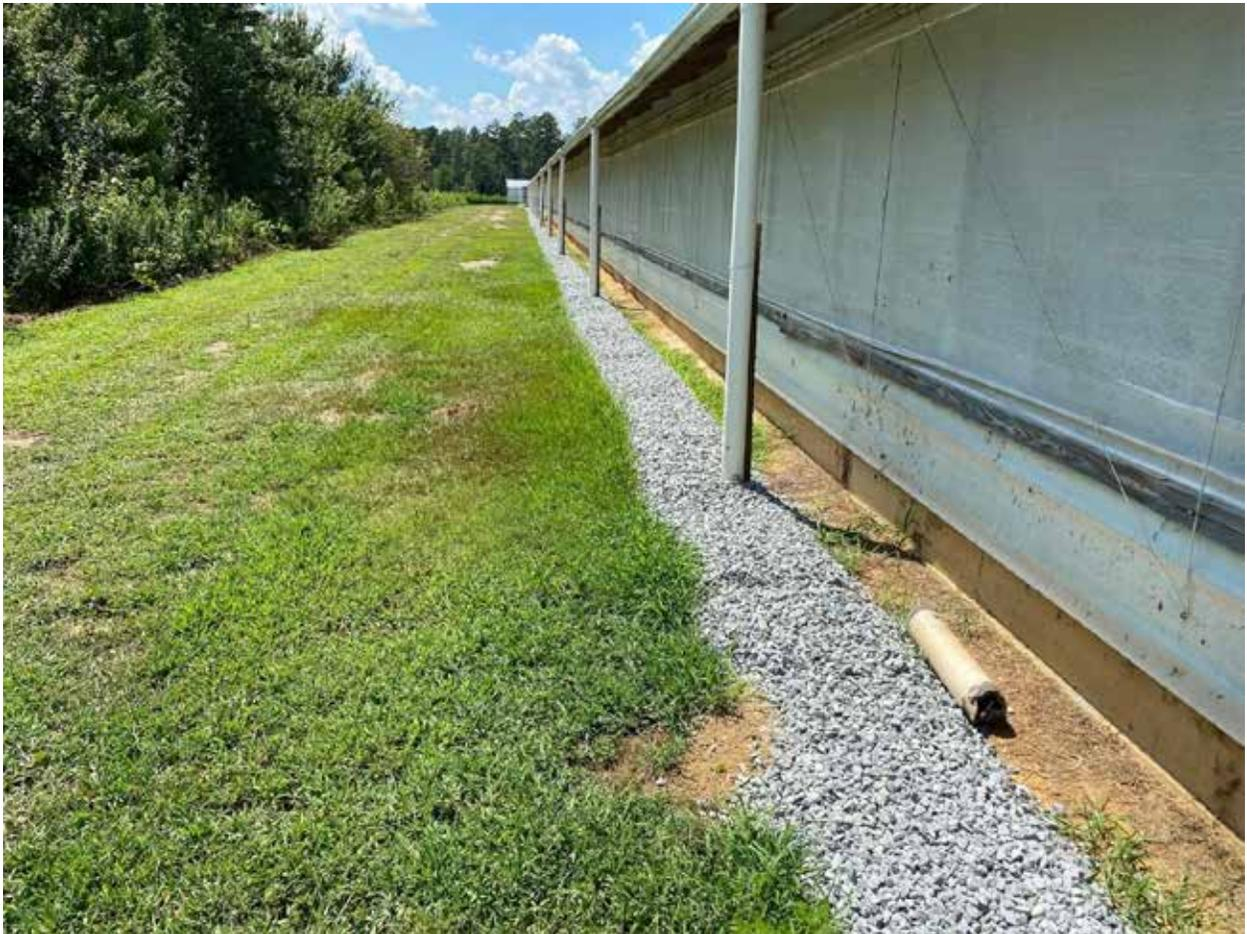
*Roof Runoff Structures are installed to prevent erosion around animal agriculture operations.*
