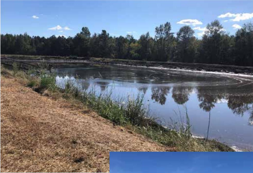
*Inactive Animal Waste Lagoons are agitated by stirring up the solids into a slurry prior to land application*
